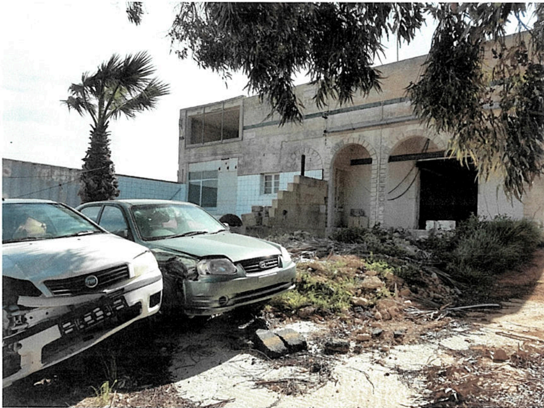
Fig. 01 ; Existing state of Slaughter house
