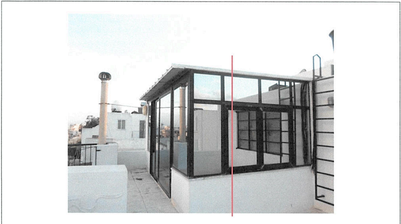
Photo 1: The structure in question ( marked in red is approximate to the required recess ). Note the temporary structure definition may only be applied from the blockwork plinth upwards.
