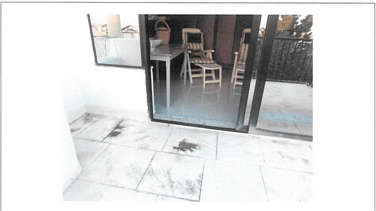
Photo 4: Elevation of Room – a 1m recess would reduce use of conservatory. Note the removal to the door sill, would disrupt the existing waterproofing works.
